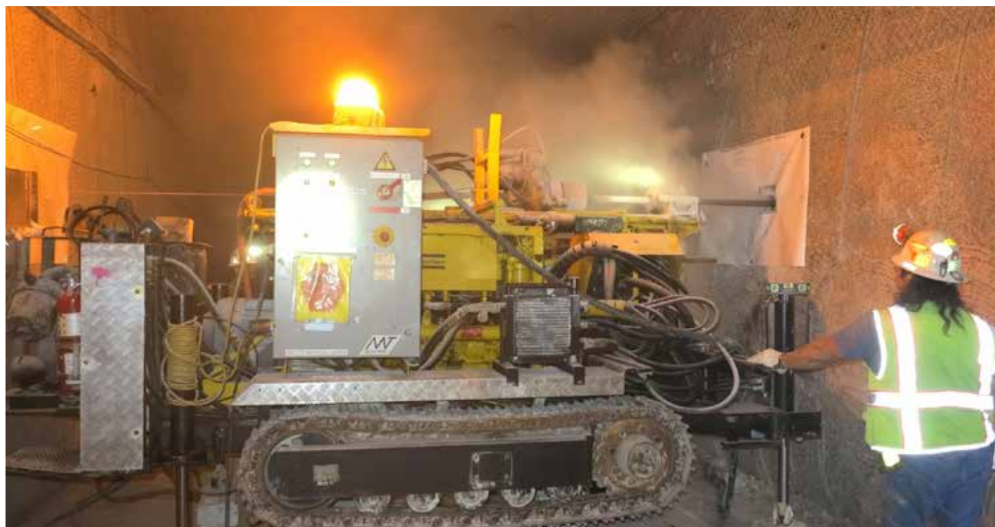
Figure 2.8) A borehole is drilled into the wall of the WIPP for experimental purposes. Source: Kristopher Kuhlman, Sandia
