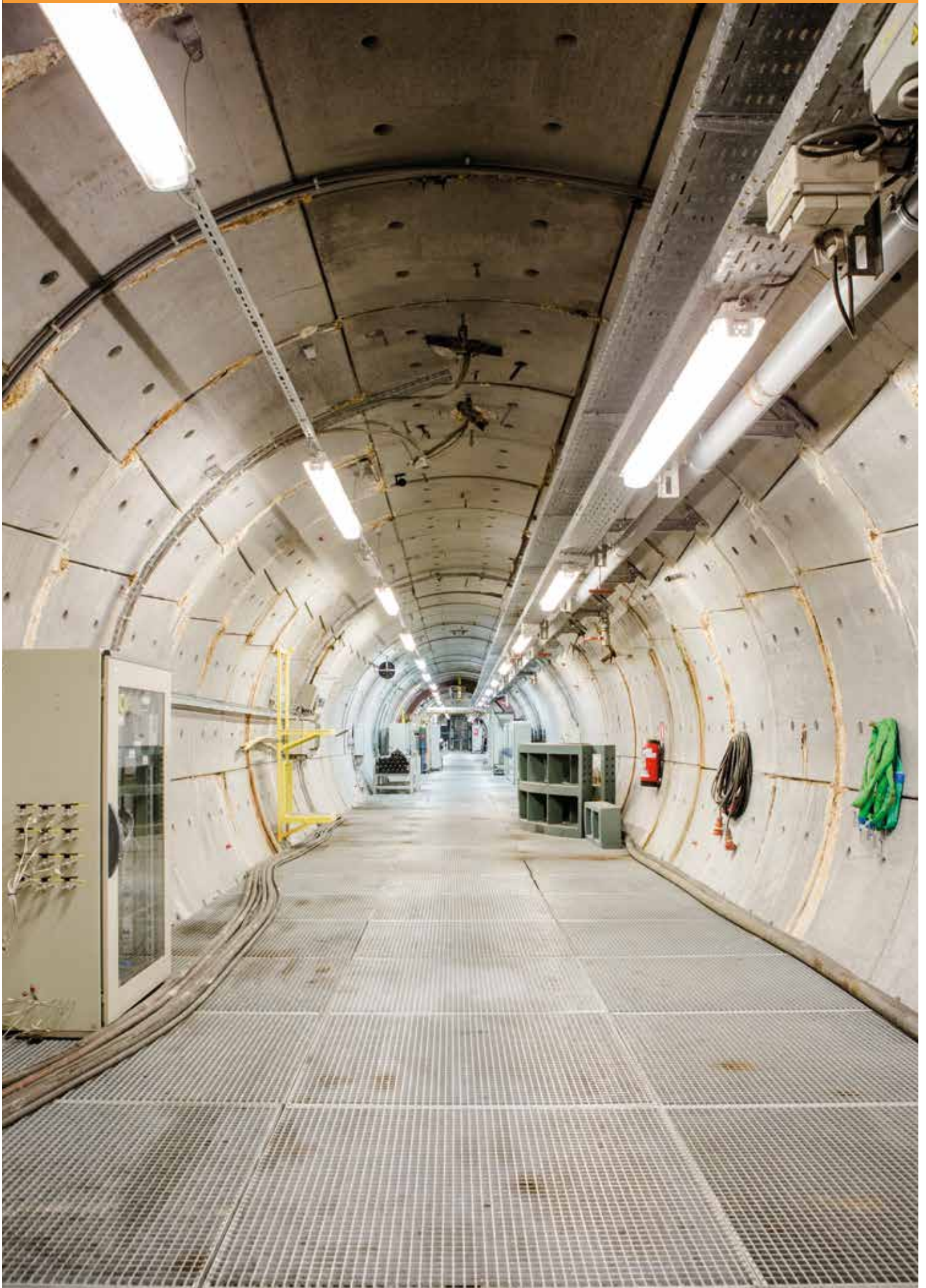
A concrete liner as an engineered construction for an underground facility in poorly indurated clay (Boom Clay). The facility remains dry by ventilation. Source: EIG EURIDICE.
